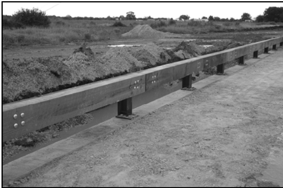
Figure 41. Traffic Side View of Tubular Steel-Backed Timber Bridge Rail
