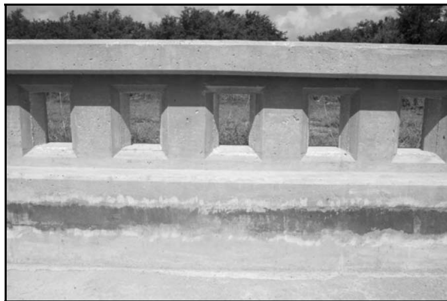
Figure 51. TxDOT F411 Bridge Rail
